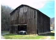
parent reason for that shape. This barn is sided with vertical boards in such a manner as to provide long, tall vent doors of one or two boards wide on metal hinges, to be opened as needed for increased air flow for the air curing of the tobacco. This farm sits in the Big Creek valley and was part of the Gaither Shelton farm.
