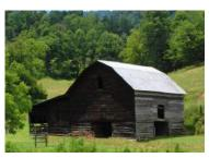
coincided with the availability of a new roofing material, metal sheet roofing, which began to replace the standard roofing material — split oak wood shingles, after WWI. The barn is also a quasibank barn with a high bank behind connected by a log bridge to the road above. The log cribs are set upon large square-hewn wood sills on field stone piers. Two additions were added at different times on the south side, as additional hanging sheds were needed for air-curing burley tobacco.
